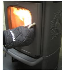
8. Once the new fuel has taken, adjust the secondary air amount to the desired setting; optimal combustion will continue until glowing charcoals are produced.
