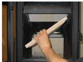
5. Lift the upper baffle out of its holder and tilt it out.
