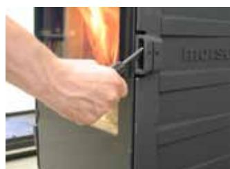
5. Re-stoking should normally be carried out while embers still remain. Distribute the embers in the bottom, ensuring that most of them are at the front of the stove.
