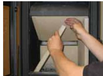
2. Tilt one of the side brick panels and remove it.
