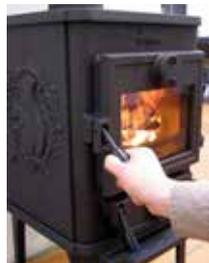
4. When the chimney is warmed through after 5-10 minutes, the door should be closed. A suitable ember bed will be formed after a further 15-20 minutes.
