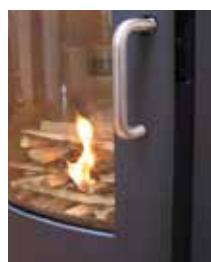
4. When you can see that the chimney is hot enough to draw (after 5 - 10 minutes), close the door. If all the necessary conditions are met, a thick layer of embers will have been formed in the combustion chamber after another 15 - 20 minutes, and there will be a high temperature in the combustion chamber, which is necessary in order to be able to continue the combustion.
